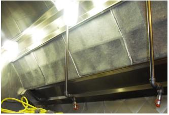
Program was initiated in the Fall of 2012. Grease Lock filters were installed in Chili's too and Popeye's in an effort to reduce residual airborne grease from entering the exhaust system and spilling grease on the roof. With the installation of the filters, we have reduce daily cleanings of the standard baffle filters, significantly reduced airborne grease from the exhaust, and reduced oil residue build up on the roof.
