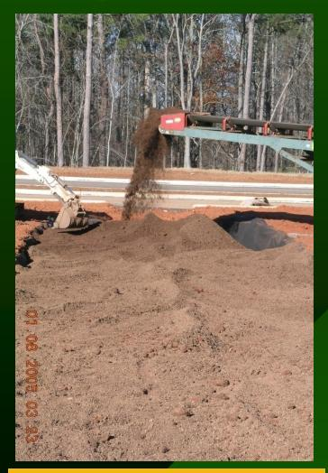
Conveyer or Blow Soil Into Place to Alleviate Over-Compaction
