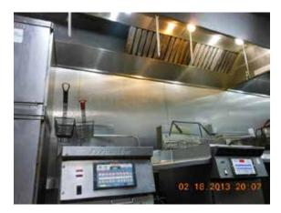
Hood # 1 and Baffle Grease Filters (# 0338)
